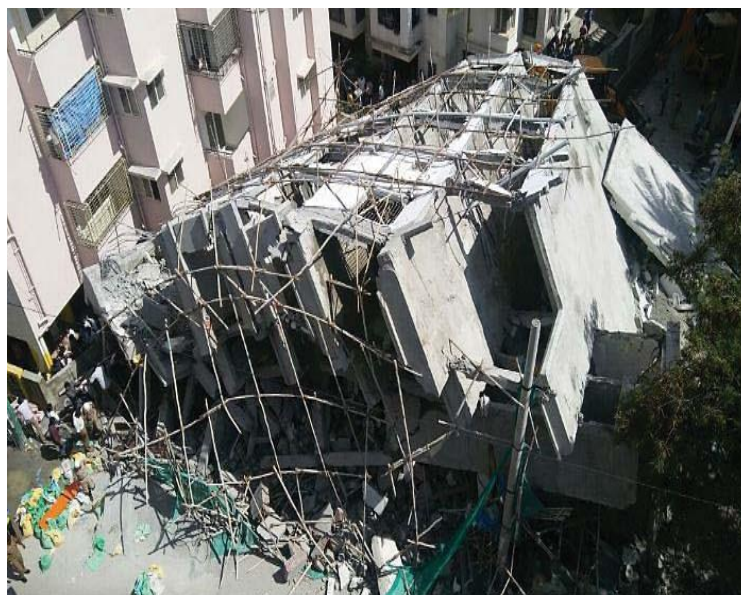
Figure 3 Building collapse at Bangalore, India (2016)
