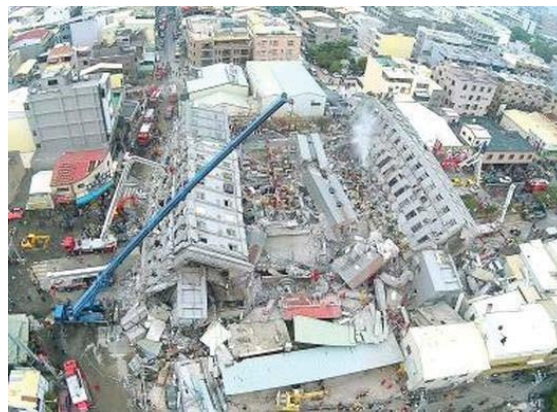
Figure 2 Weiguan Golden Dragon building collapse due to earthquake (2016)
