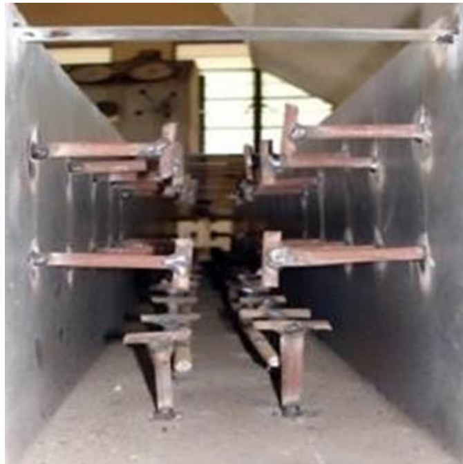
Figure 2 Trough Section of CSCC Beam
