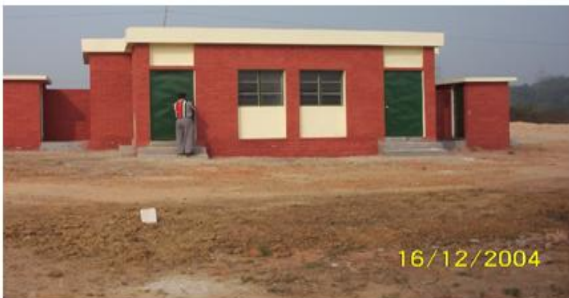
Figure 2: A VAMBAY HOUSE AT DURGAPUR.
