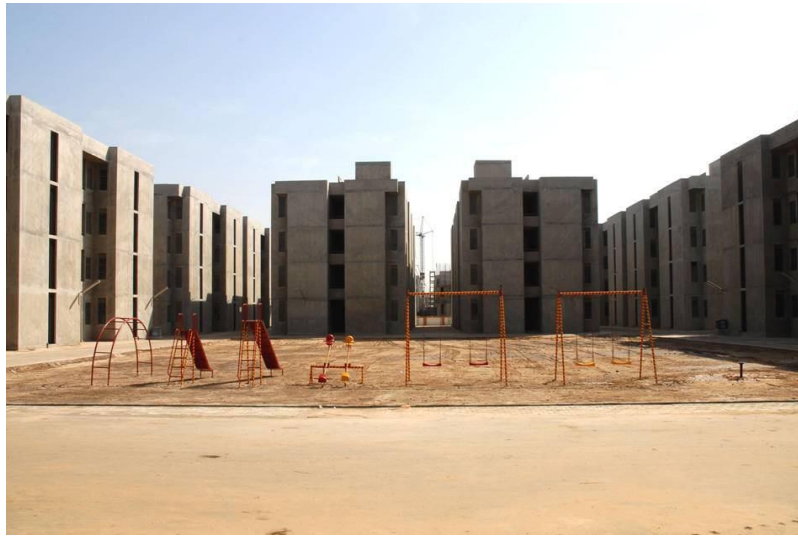
Figure 5: A tot inside the heart of the housing of Ahmedabad Municipal Corporation.
