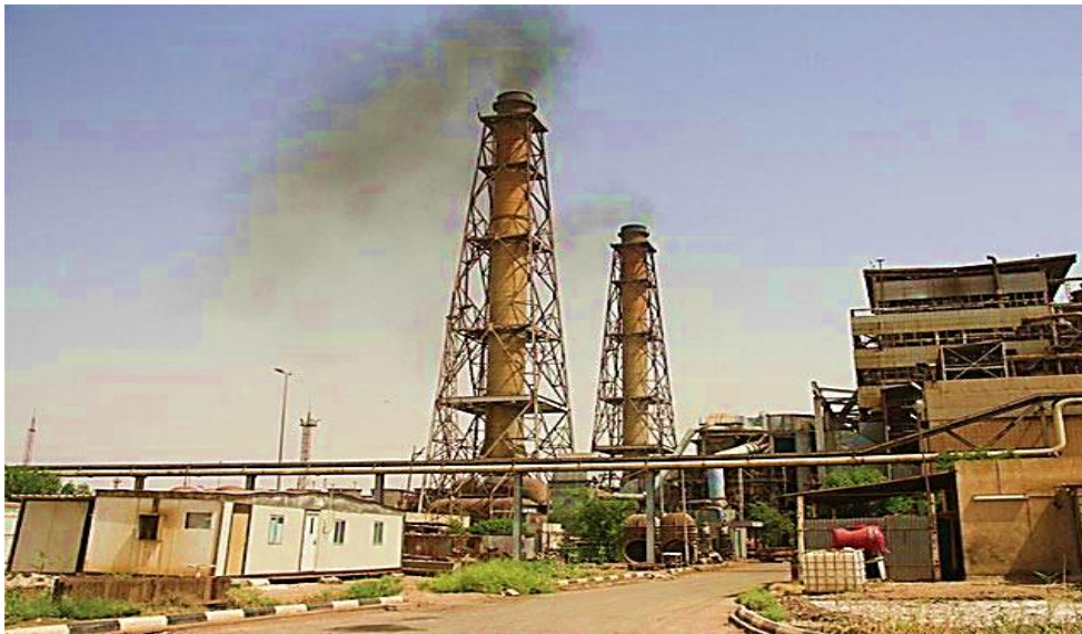
Figure (2) View of the chimneys of Nassiriya Thermal Power Station (Iraq, Nassiriya City) [11].
