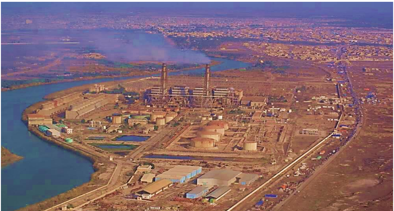
Figure (1) Nassiriya Thermal Power Station (Iraq, Nassiriya City) [10].
